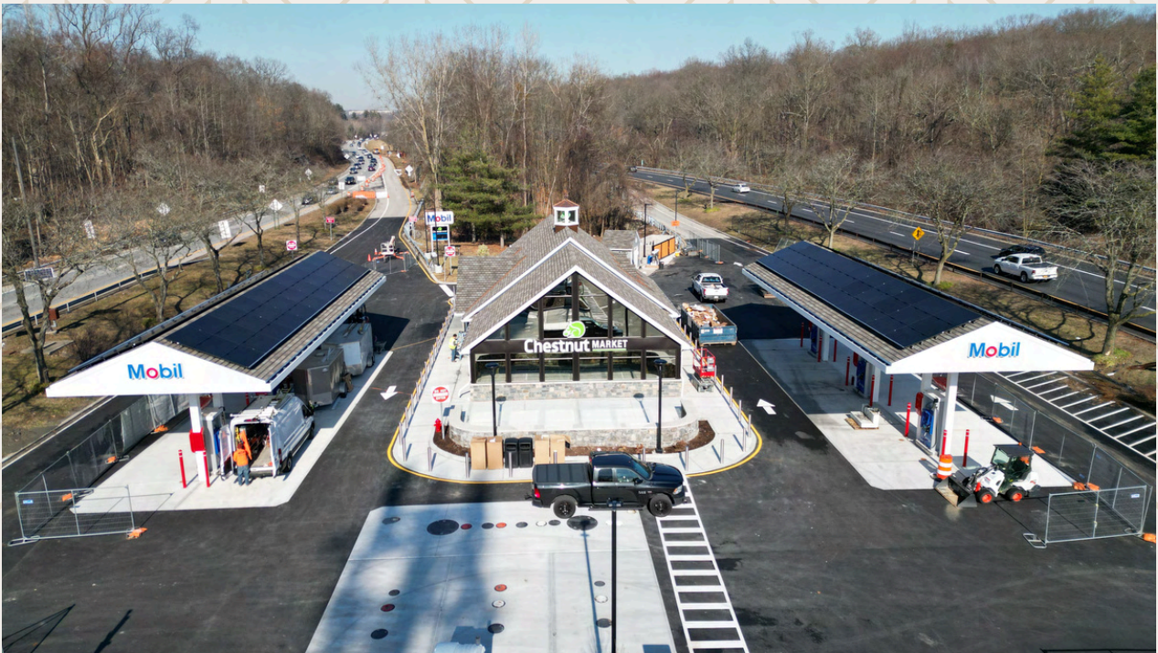
CPD Energy Group-Hutchinson River Parkway
